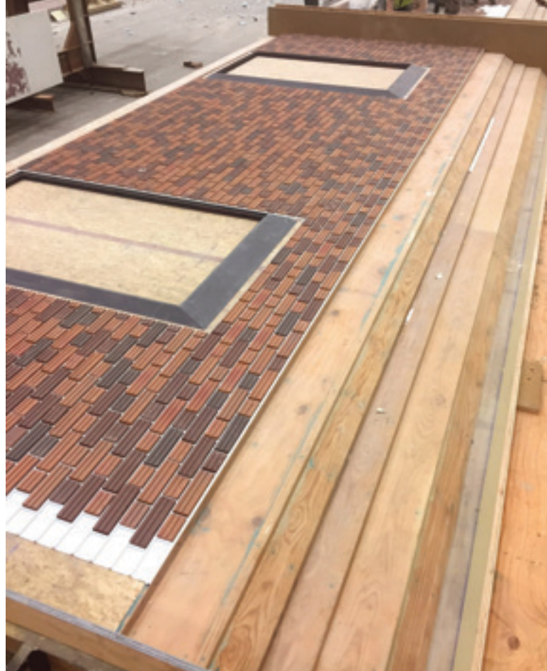
The casting of the wall panels for the Pioneer Hall project featured inset brick surrounding the 3-D printed blockouts that created the window shapes. Photo: Wells Concrete.
