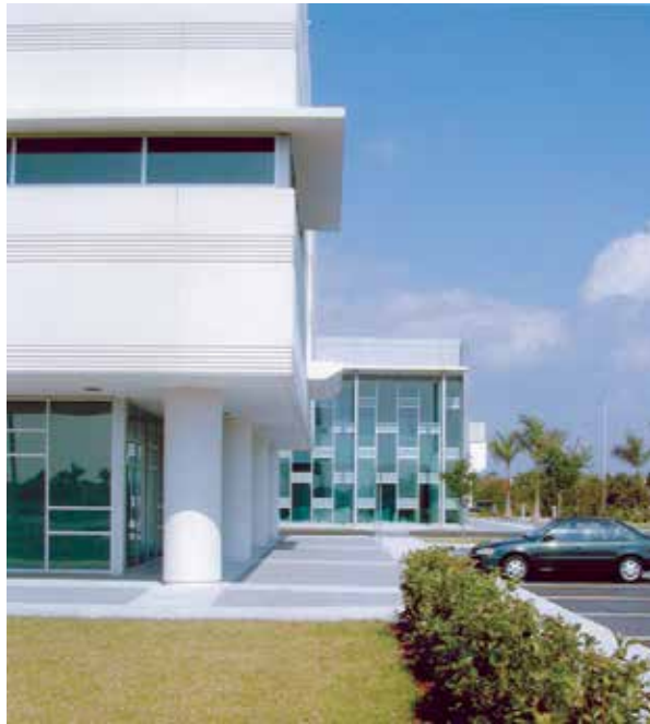
Figure 7 High-reflecting (usually light-colored) surfaces help mitigate urban heat islands. Cape Coral City Hall, Cape Coral, Fla.; Architect: Spillis Candela/DMJM. (Courtesy Spillis Candela DMJM)
