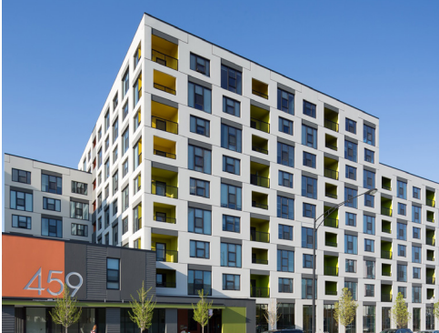
Terrace 459 at Parkside of Old Town Chicago, IL. Photo: David Shalilol, and Landon Bone Baker Architects.
