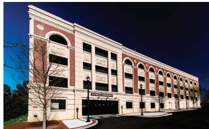
Alpharetta City Center Parking Garage, Alpharetta, GA. Photo: George Spence.
