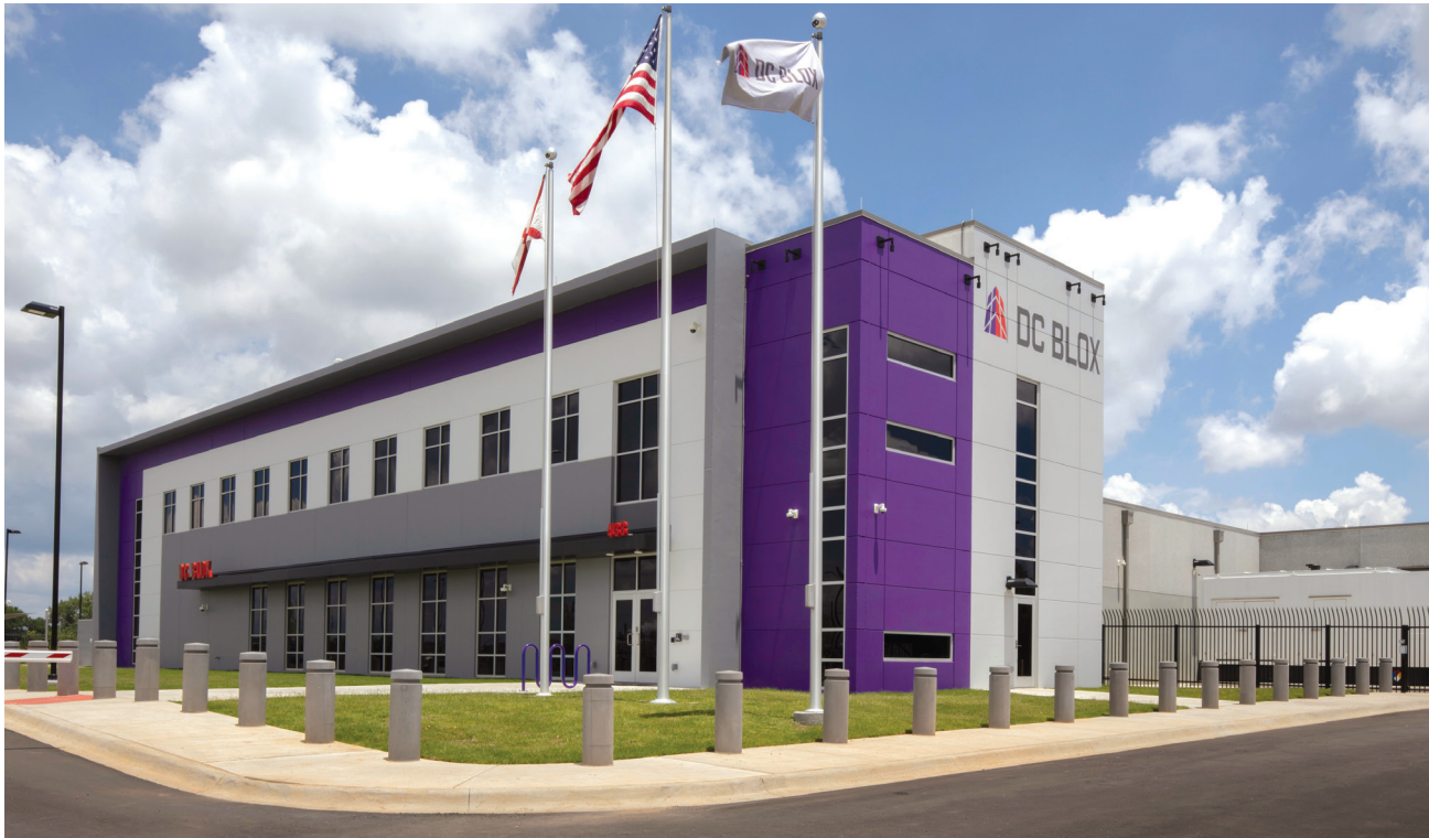
DC Blox Data Center, Birmingham, AL. Photo: DC Blox.
