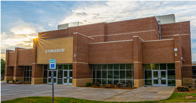
Smithfield Middle School Gymnasium Addition and Storm Shelter, Haltom City, TX. Photo: Eric Childs, Key Construction
