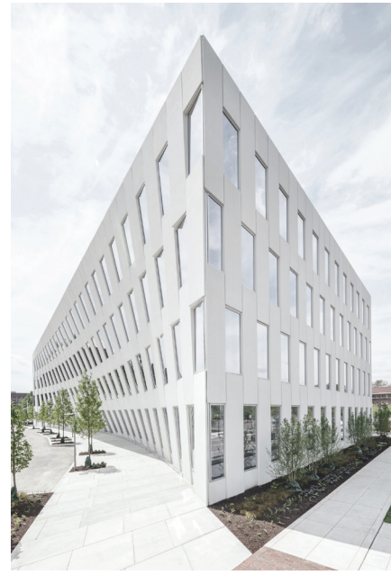
1200 Intrepid Building, Philadelphia, PA. Photo: Bjarke Ingels Group.
