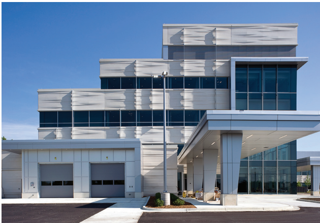
Marshfield Clinic Health System Hospital and Cancer Center, Eau Claire, WI. Photo: Gage Brothers.
