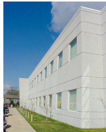
McQueary Family Health Science Hall, Missouri State University, Springfield, MO. Photo: Prestressed Castings Co.
