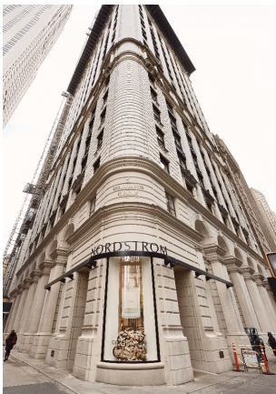
Nordstrom NYC Flagship Store, New York, NY. Photo: Gate Precast Company.
