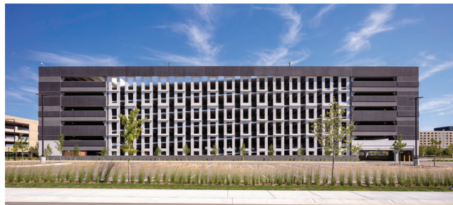
Health Partners Bloomington Parking Structure, Bloomington, MN. Photo: McGough Construction Co., Inc., Wells Concrete.
