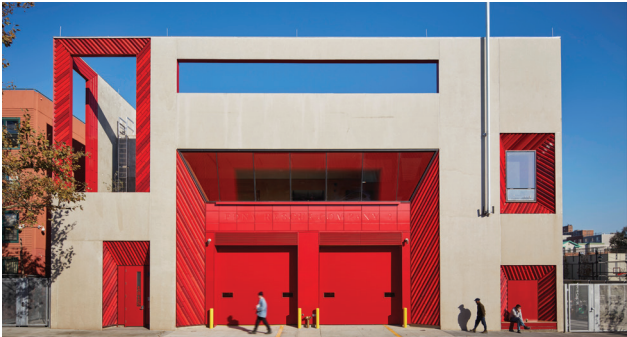
Fire Department of New York Firehouse Rescue #2, Brooklyn, NY. Photo: High Concrete Group.
